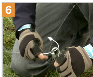
6 Loop guy wire through Quick Link
