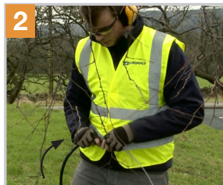
2 Thread guy wire through rubber sleeve sleeve
