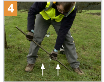
4 Activate Anchor by pulling the wire upwards
