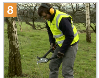
8 Tension at ground level to straighten tree
