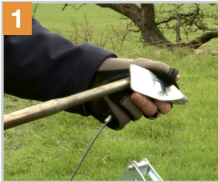
1 Insert Drive Rod into the Terra-Lock™ Anchor
