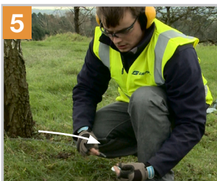
5 Thread guy wire through the second tensioner at ground level
