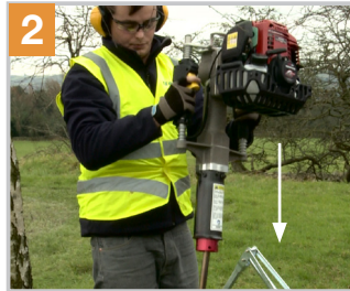
2 Drive the Anchor until the loop is just above ground level
